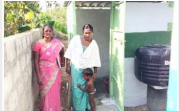
Construction of Household Toilets
